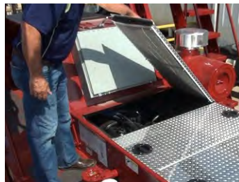
Lightweight Deck Lids and Easy Access to Heavy Duty Circuit Breaker Panel
