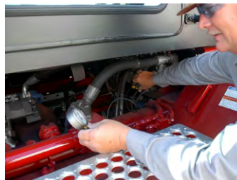
Service & Inspection from Ground Level
